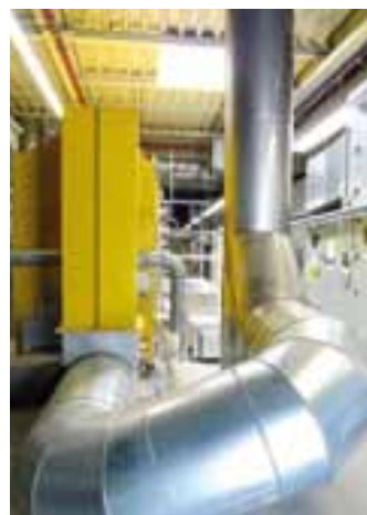
Ducts between the TRA and chimney, part of the impressive in-plant technology centre
